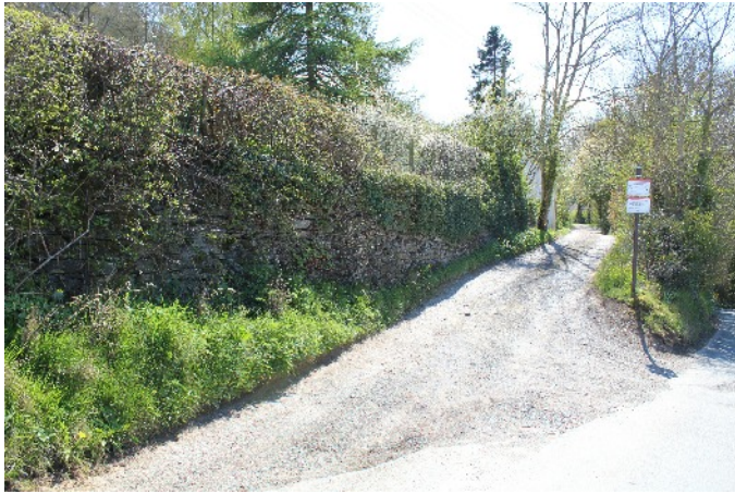
Site of the level crossing where the trackbed crossed the Bontuchel-Rhewl lane. This crossing is visible bottom centre in the LIDAR image below.
