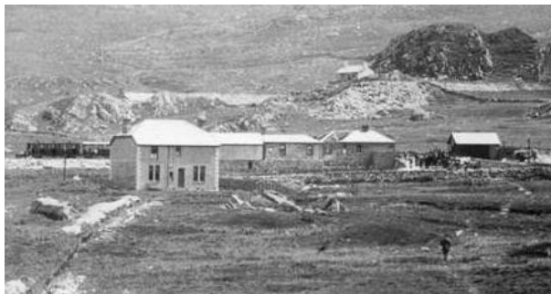
An enlarged detail from a Carl Norman image - No. 7106 - showing building extension work in progress at Rhyd-ddu.
