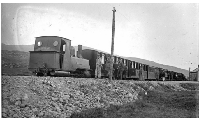
The 'exit embankment' from the north-west - Arch 4397
