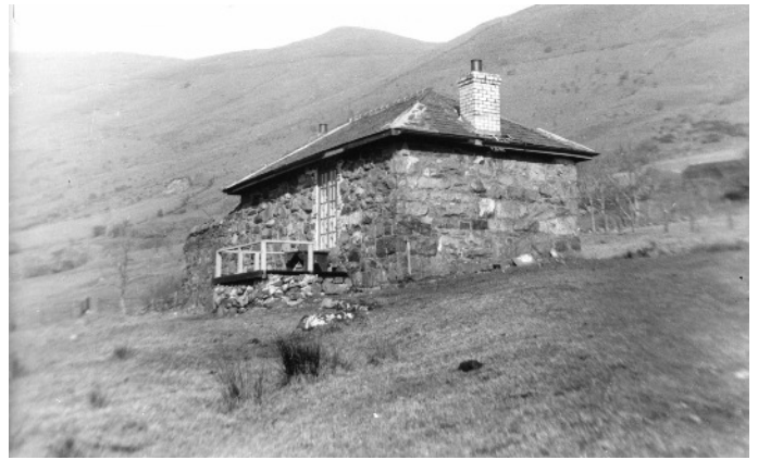
Snowdon Ranger station building - Arch 4575 - Bill Rear - 1948
