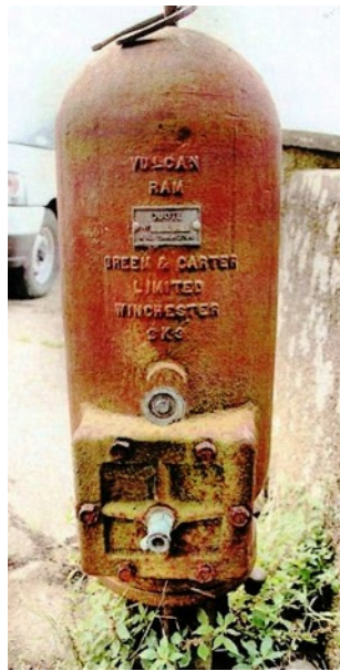
Left: JK 'fettling' the valve assembly from the hydraulic ram pump whose compression chamber is seen in full in the centre image. Right: the original water supply line from Nant Cwmcloch to the Beddgelert water tower.
