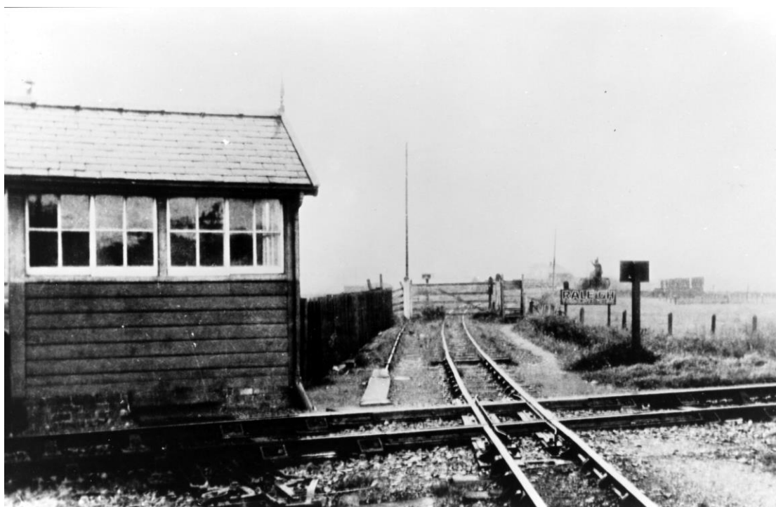
6. above From the south side looking north, again showing the 1928 GWR crossing fitment. The rodding runs to the north and south trap points can be seen. Compare with photos 3 and 5. There is an advertising sign (for Raleigh bicycles) alongside the WHR track, short of the gate. Note the stile by the right-hand side of the gate. Photo by W D Miller, 1932
