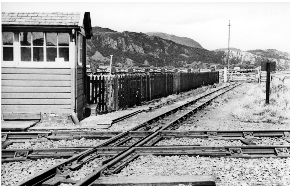
9. above The crossing from the south: another useful comparison with photo 3 of a decade earlier (the piece of fence and rodding run cover are in place!) and photos 5 and 6. The 1928 crossing fitment – in bridge rail and angle-iron style check rails – is clearly shown. Photo by F C LeManquais, 11 August 1934.
