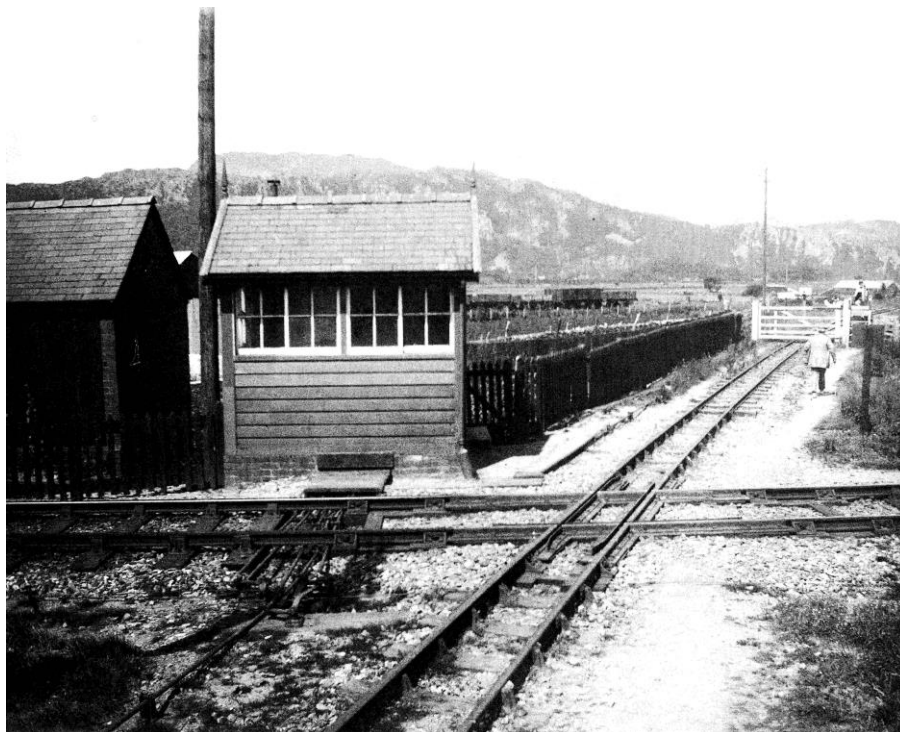
5. above From the south side looking north, showing the 1928 GWR crossing fitment. The rodding runs to the north and south trap points can be seen. Compare with photos 3 and 6. This appears to be a passenger walking to the north platform (is there another climbing the stile by the gate across the line? it looks as though the photographer was on the equivalent stile on this side of the line) which was brought into use from the 1929 season to avoid WHR passenger trains having to traverse the crossing. The date was a Monday during the last week of the pre-season thrice weekly service on the WHR. The advertising sign (for Raleigh bicycles) shown in photo 6 does not yet appear to be in place. The wagons beyond the box are on the standard gauge Beddgelert Siding. The end of the crossing cottage is to the left of the box. Photo by Edward Wallis, 1 July 1929
