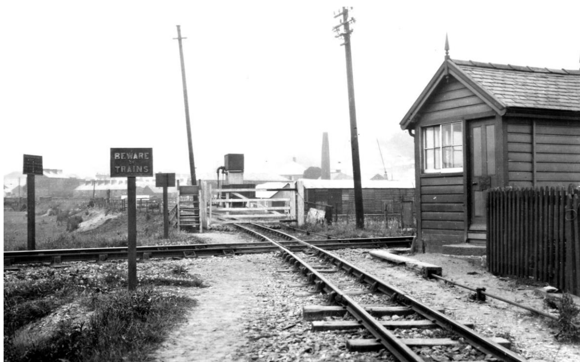
4. above From the north side looking south, showing the new GWR crossing fitment. The New station's water tower is prominent above the gate. Note post and wire fencing opposite the box (on the GWR's down side) instead of white fence in photo 1. The left hand telegraph pole is that in photo 2, the right hand one is that in photo 1. Locomotive Publishing Co. photo no. 1663 (later 77880) had usually been dated summer 1928 but it must post-date the relaying of the crossing fitment on 28 October 1928
