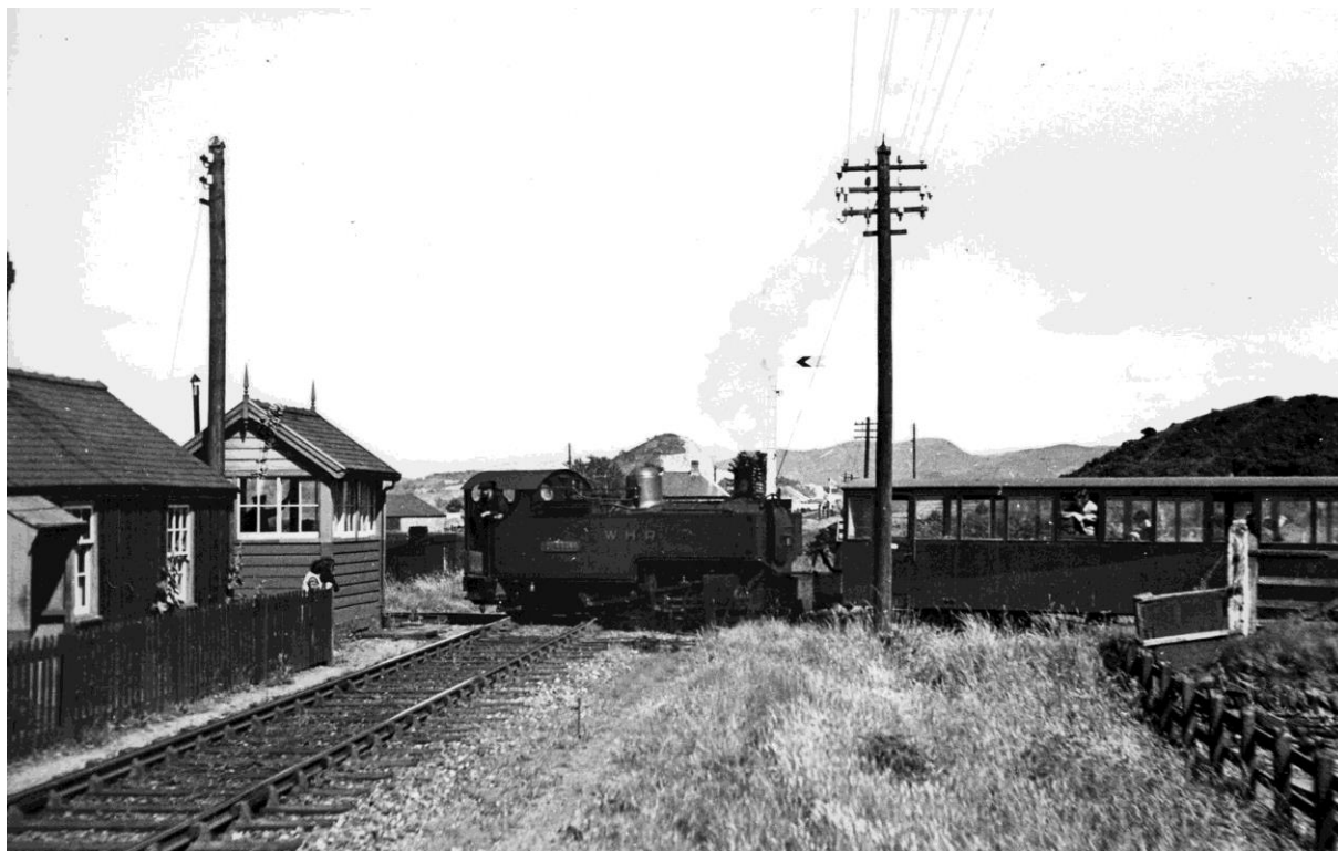
11. above The crossing from the west, with Russell on a Down train, providing another comparison with photo 1 of an earlier decade. Looking in the opposite direction from photo 10, it shows the east corner of the crossing cottage, left, as well as the box. The GWR Down stop signal, protecting the WHR train, is obscured by steam above Portmadoc's (formerly East box) Distant which can be seen. Photo by Stanhope W Baker, 8 July 1936.
