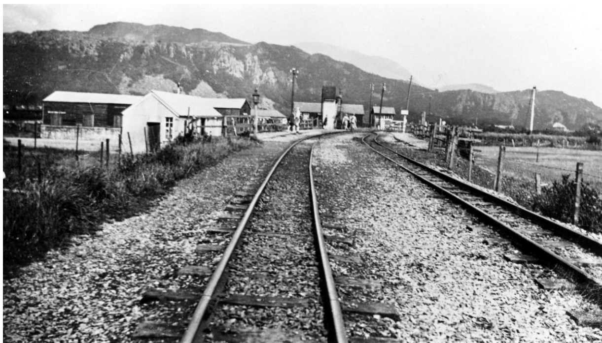
12. above A view from the south side: a photograph of the 1923 station with no train in the way! It thus provides a useful panorama of the crossing cottage (behind the WHR water tower), box (behind south gate), GWR Down Stop signal (extreme right) – and various telegraph poles that dot the landscape! Photo by Charles Loch Mowat, most likely summer 1926.
