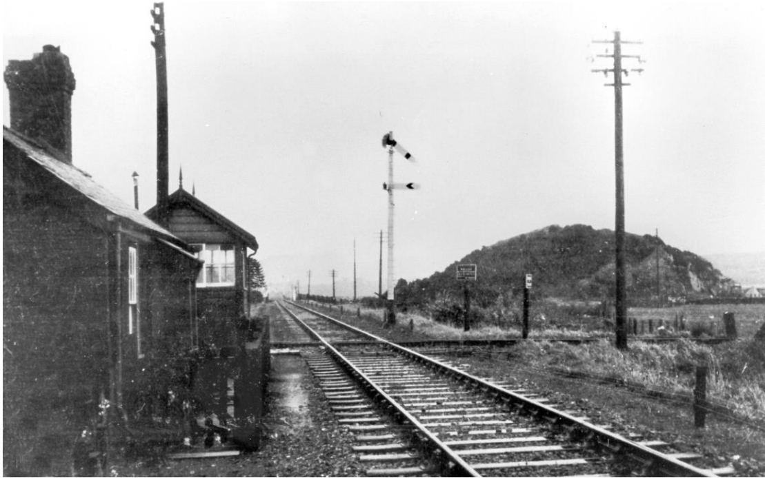
7. above . The crossing from the Gelert's Farm occupation road crossing, looking east towards Minffordd, with the cottage extreme left and the box beyond. The crossing's Down stop signal (with Portmadoc's fixed distant arm beneath it) is prominent – as is the hill, Ynys Cerrig-duon, mentioned in the A&WC Acts. This picture shows clearly how the Cambrian line was built north of that rock, rather than south of it as envisaged in the plan on page 2. The 1923 New station is off to the right of the picture. The telegraph pole on the right is that shown in photo 1. Only a close scrutiny reveals evidence of Traethmawr road crossing in the distance. Photo by W D Miller, presumed to be 1932 (contemporary with photo 6)
