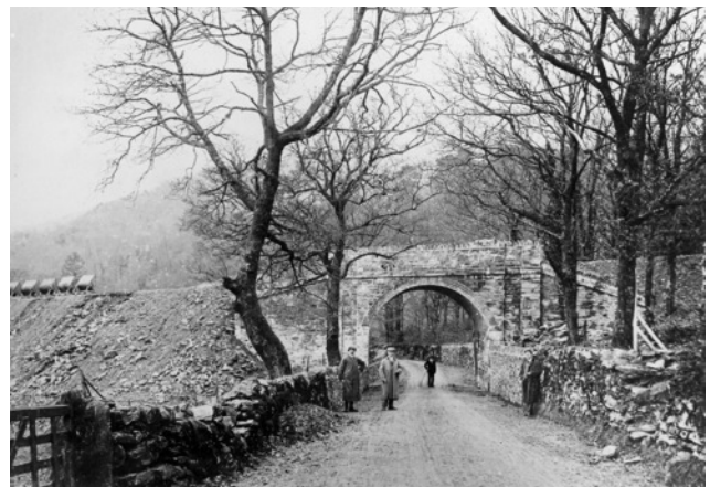
The 'Bridge to Nowhere', and the embankment down to the proposed PBSSR Glaslyn crossing, under construction - 1905 - WHR 203
