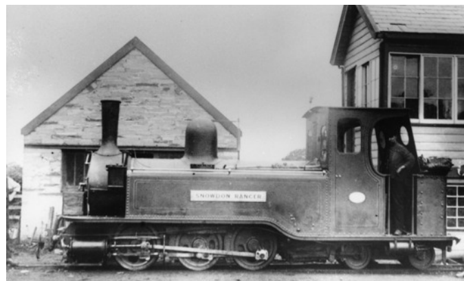
Two pictures of Snowdon Ranger at Dinas - Top, WHR 6, credited to H.L. Hopwood, June 1909 - Bottom, Arch 3180, also Hopwood, also June 1909.
