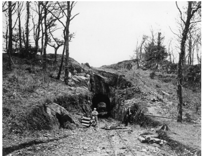
The Goat Tunnel excavations from the other end, looking towards Beddgelert Station - ca. 1905 - WHR 200
