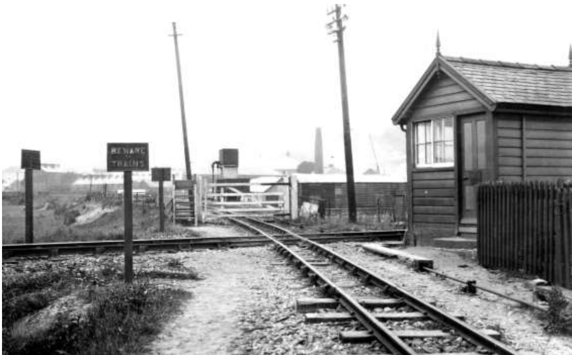
4. above From the north side looking south, showing the new GWR crossing fitment. The New station's water tower is prominent above the gate. Note post and wire fencing opposite the box (on the GWR's down side) instead of white fence in photo 1. The left hand telegraph pole is that in photo 2, the right hand one is that in photo 1. Locomotive Publishing Co. photo no. 1663 (later 77880) had usually been dated summer 1928 but it must post-date the relaying of the crossing fitment on 28 October 1928
