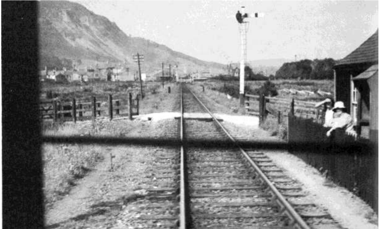
10. above The right foreground is the west corner of Croesor Crossing cottage with the road access (occupation crossing) to what is now Gelert's Farm beyond. The photo was taken from the Pickering Brake-Composite no. 8 in a Down WHR train at the moment of crossing the GWR. The Stop signal – at Danger – protects the train from Up GWR trains. The crossing gates at Portmadoc East can be seen in the distance, closed across the GWR. Photo by H F Wheeler, 8 August 1935.
