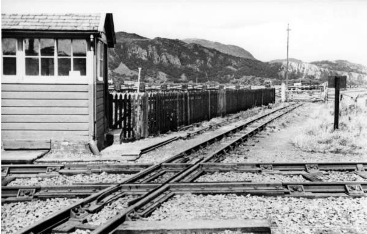
9. above The crossing from the south: another useful comparison with photo 3 of a decade earlier (the piece of fence and rodding run cover are in place!) and photos 5 and 6. The 1928 crossing fitment – in bridge rail and angle-iron style check rails – is clearly shown. Photo by F C LeManquais, 11 August 1934.
