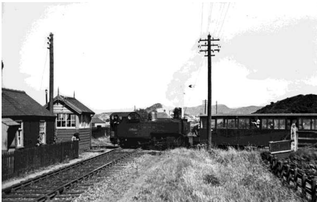
11. above The crossing from the west, with Russell on a Down train, providing another comparison with photo 1 of an earlier decade. Looking in the opposite direction from photo 10, it shows the east corner of the crossing cottage, left, as well as the box. The GWR Down stop signal, protecting the WHR train, is obscured by steam above Portmadoc's (formerly East box) Distant which can be seen. Photo by Stanhope W Baker, 8 July 1936.
