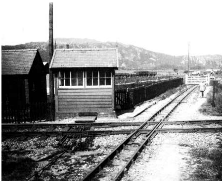
5. above From the south side looking north, showing the 1928 GWR crossing fitment. The rodding runs to the north and south trap points can be seen. Compare with photos 3 and 6. This appears to be a passenger walking to the north platform (is there another climbing the stile by the gate across the line? it looks as though the photographer was on the equivalent stile on this side of the line) which was brought into use from the 1929 season to avoid WHR passenger trains having to traverse the crossing. The date was a Monday during the last week of the pre-season thrice weekly service on the WHR. The advertising sign (for Raleigh bicycles) shown in photo 6 does not yet appear to be in place. The wagons beyond the box are on the standard gauge Beddgelert Siding. The end of the crossing cottage is to the left of the box. Photo by Edward Wallis, 1 July 1929
