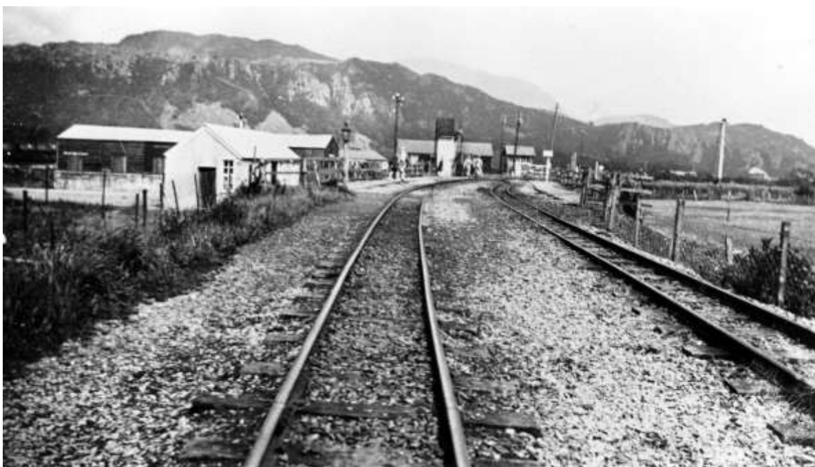
12. above A view from the south side: a photograph of the 1923 station with no train in the way! It thus provides a useful panorama of the crossing cottage (behind the WHR water tower), box (behind south gate), GWR Down Stop signal (extreme right) – and various telegraph poles that dot the landscape! Photo by Charles Loch Mowat, most likely summer 1926.
