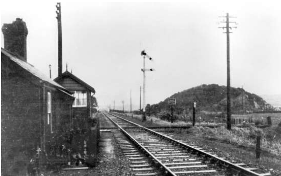
7. above . The crossing from the Gelert's Farm occupation road crossing, looking east towards Minffordd, with the cottage extreme left and the box beyond. The crossing's Down stop signal (with Portmadoc's fixed distant arm beneath it) is prominent – as is the hill, Ynys Cerrig-duon, mentioned in the A&WC Acts. This picture shows clearly how the Cambrian line was built north of that rock, rather than south of it as envisaged in the plan on page 2. The 1923 New station is off to the right of the picture. The telegraph pole on the right is that shown in photo 1. Only a close scrutiny reveals evidence of Traethmawr road crossing in the distance. Photo by W D Miller, presumed to be 1932 (contemporary with photo 6)
