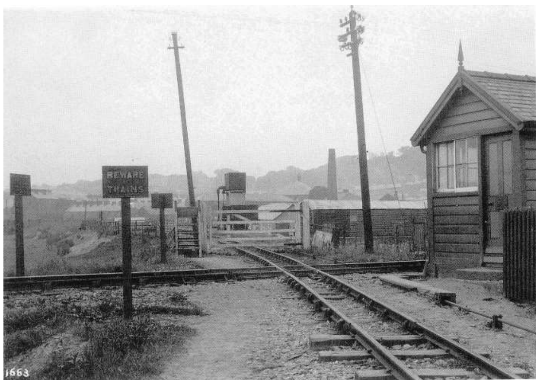
4. above From the north side looking south, showing the new GWR crossing fitment. The New station's water tower is prominent above the gate. Note post and wire fencing opposite the box (on the GWR's down side) instead of white fence in photo 1. The left hand telegraph pole is that in photo 2, the right hand one is that in photo 1. Locomotive Publishing Co. photo no. 1663 (later 77880) has, until now, usually been dated summer 1928 but it must post-date the relaying of the crossing fitment on 28 October 1928
