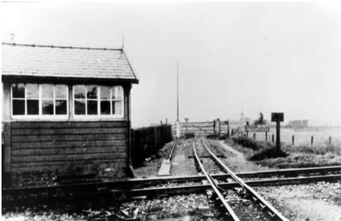
6. above From the south side looking north, again showing the 1928 GWR crossing fitment. The rodding runs to the north and south trap points can be seen. Compare with photos 3 and 5. There is an advertising sign (for Raleigh bicycles) alongside the WHR track, short of the gate. Note the stile by the right-hand side of the gate. Photo by W D Miller, 1932
