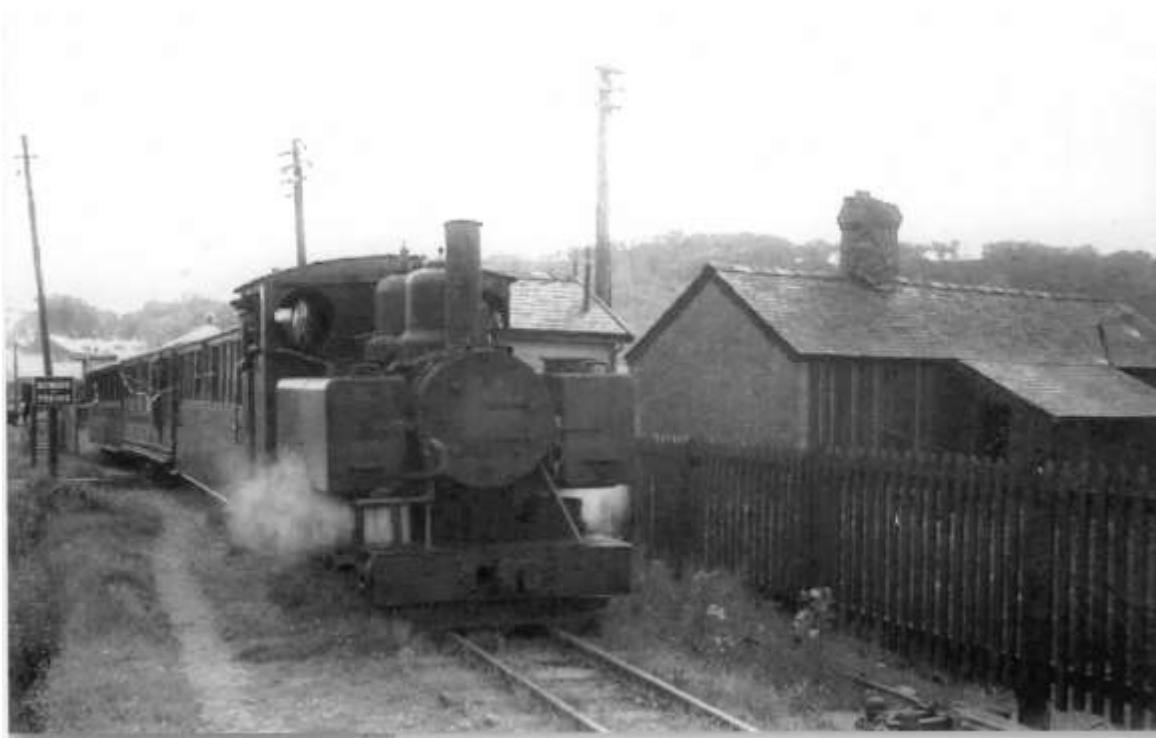
8. above Baldwin 590 on a three coach Down train. Although the crossing box is largely hidden, the crossing cottage is clear – as are three of the four telegraph poles! The bell crank (bottom right) is part of the rodding run to the north trap point. The only date offered for this photo from FR Archives is "1930s". However, the orientation of the loco puts the photo as being during the FR lease period, i.e. 1934-1936.
