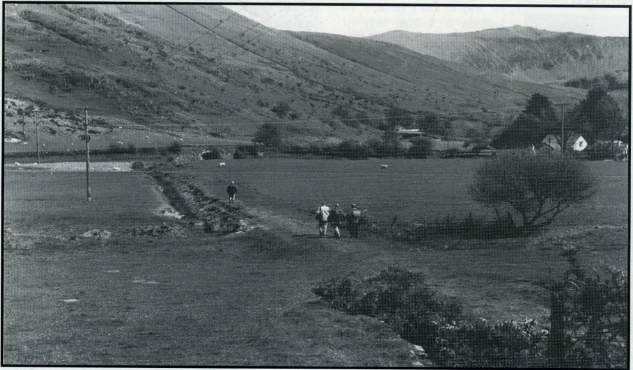
“Survey Party approaching Quellyn Lake Road bridge”
