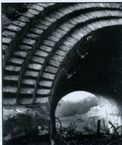
Road Over Bridge at Waenfawr D. Allan - April 1998
