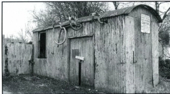
Corrugated iron "petrol store" at Dinas?
