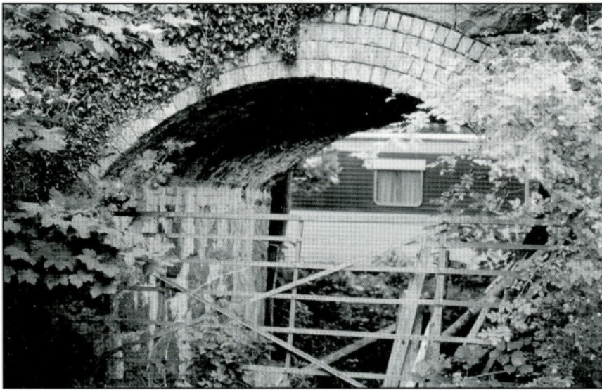
Disused bridge at Bryn Gloch. Photo D.W. Allan
