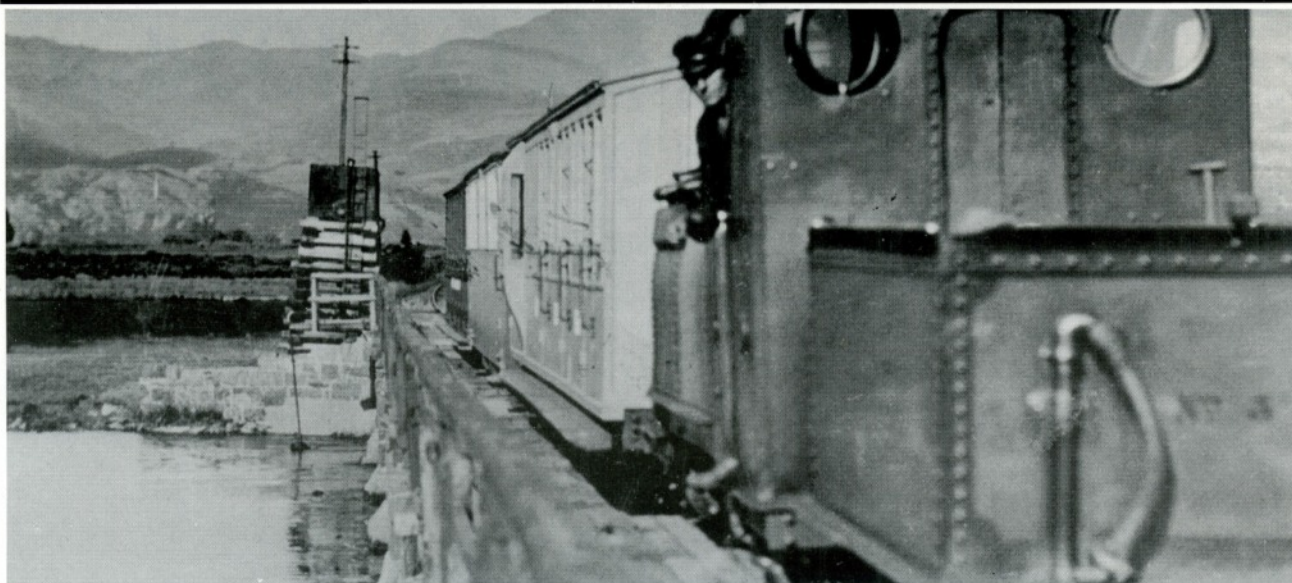
'Welsh Pony' and train crossing Pont Croesor in 1934. Note the tank feeder pipe which is under the bridge and clamped to it. Photo Roger Kidner - 1934. (Photo is much enlarged)
