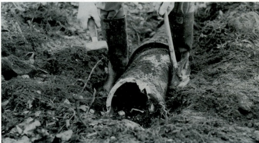
Removing an example of the buried water supply pipe. Photo - David Allan, December 1999.
