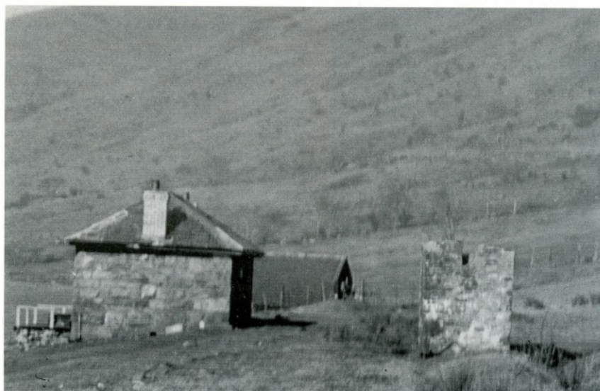
Snowdon Ranger station photographed in 1948 by Bill Rear with the remains of the water tower in the foreground.
