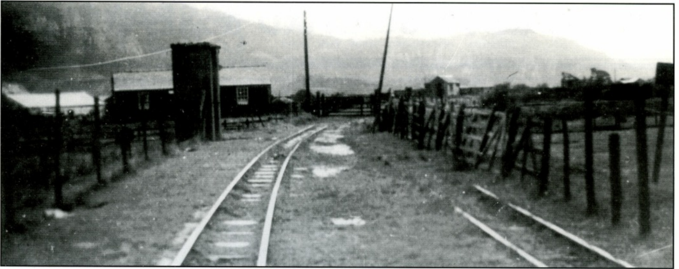
After closure - narrow gauge severed, signals gone, 'New' station still visible. (JIC Boyd collection)
