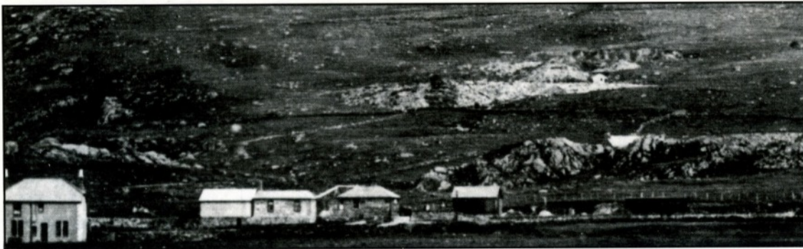
An early view of South Snowdon with work apparently going on to construct a building between the two originals. Photographer unknown.
