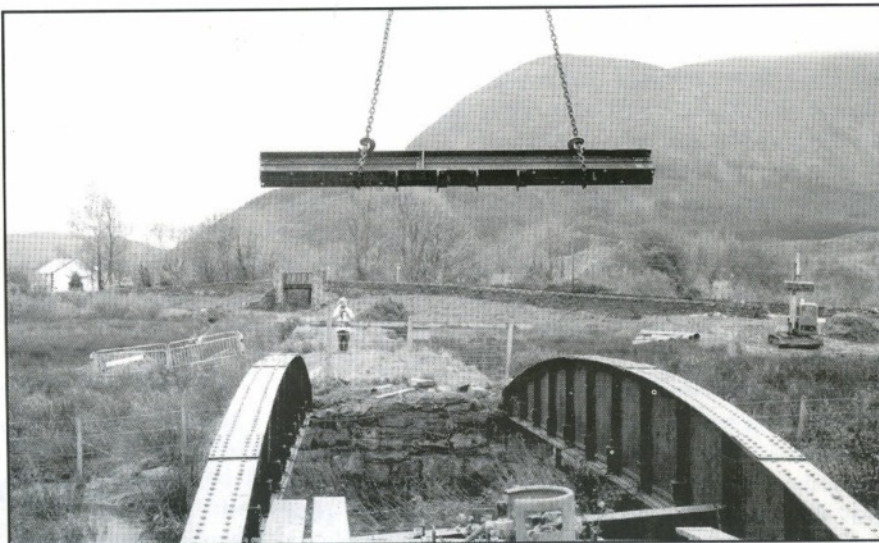
Bridge lifting in progress. Photo D.W. Allan - 2nd November 2000
