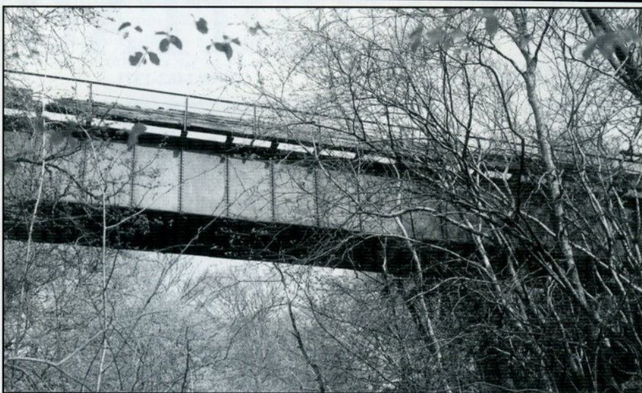
Glan yr Afon viaduct from below. D.W. Allan. - Date 30th April 1997
