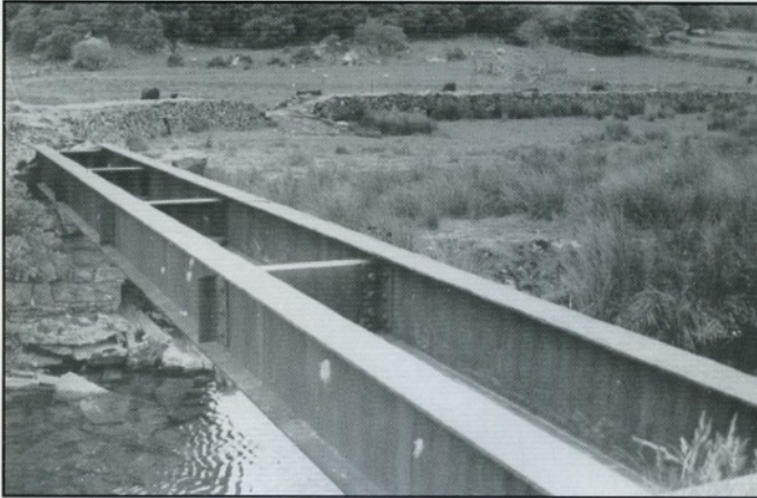
Girders over the Afon Gwyfrai which had once carried the rails to Treflan and Garreg Fawr slate quarries. Just beyond the end of the girders there was a junction with one line of track carrying straight on and the other curving sharply to the right on the slate built embankment visible in the background of the photograph
