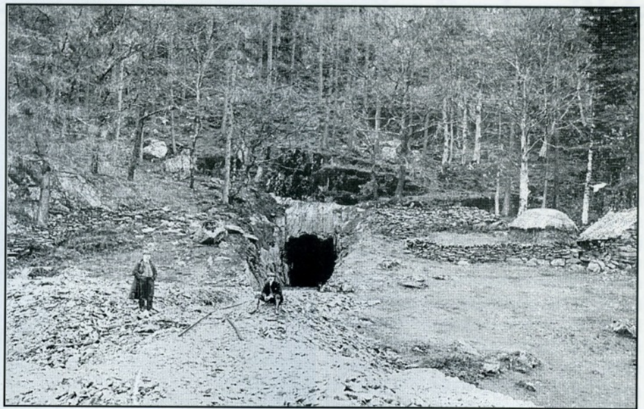
Work nearing completion at the Nantmor end of the Long Tunnel in the Aberglaslyn Pass. Photo P.G. Thomas 1906.
