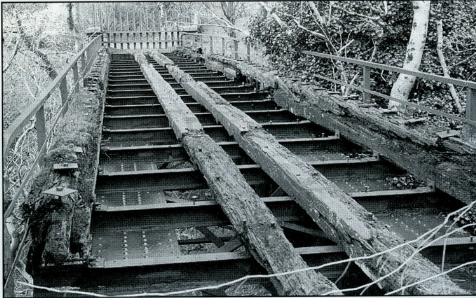
Glanrafon Viaduct 46 years later! Photo David Allan, 12th April 2000
