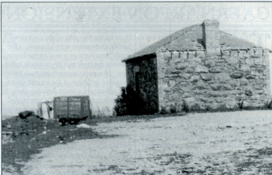
Rhostryfan station building. Date & photographer unknown
