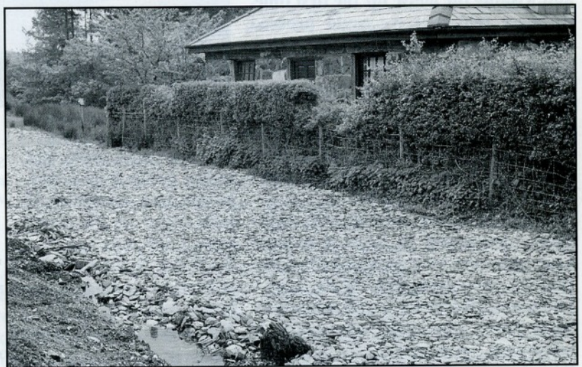
Stump of 'Home' signal (bottom centre) with Snowdon Ranger station in background.
