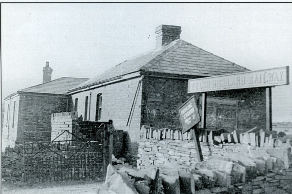
Rear of the building - note the gent's urinal flushed by the downspout! A 1939 picture by Photomatic. (Ref G36 - 16)
