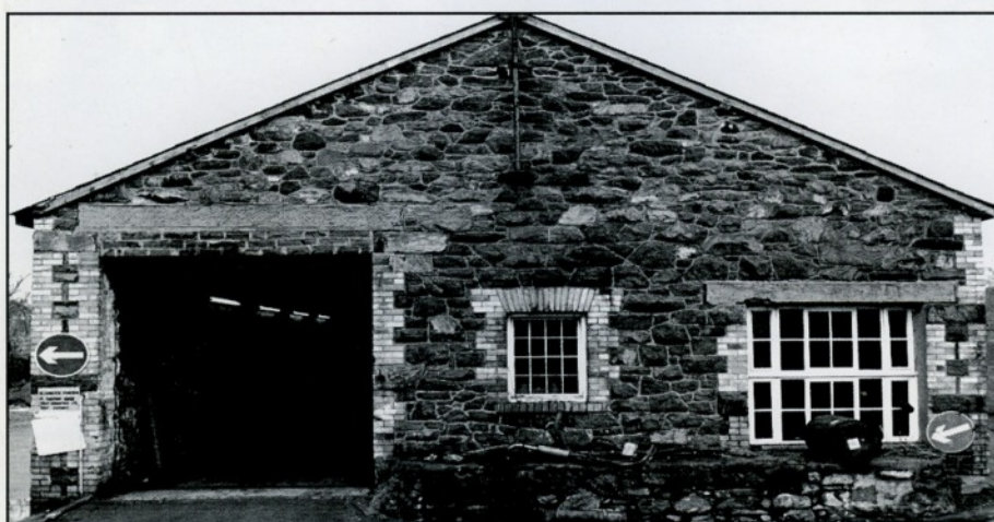
Dinas Goods Shed on 26th January 1988, Left - standard gauge entrance, centre - original NWNG window, right - narrow gauge exit, then used as a window Photo David Allan.
