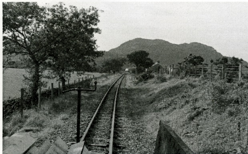
Pont Croesor extension from Gelert's Farm,, north of Cynfal. Showing how the railway was 'cut into' the Creassy embankment, The field to the left is the foot of the embankment and the top of it is to the right. D. Allan October 2006
