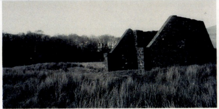
Part-built, never used accommodation bridge in the field near Gelert's Grave. Photo David Allan - 1988
