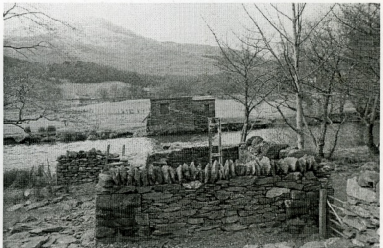
PB&SSR abortive bridge abutments over the Glaslyn, constructed 1906. Photo - David Allan
