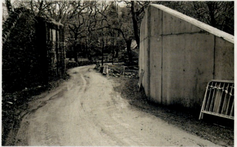
Old & new- Cwm Cloch bridge February 2007 David Allan
