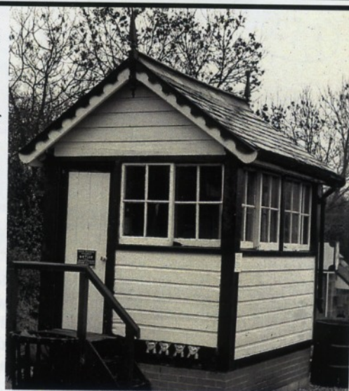
The very similar Dutton Type 4 signal box originally at Llansantffraid Crossing, seen here at the erstwhile Myddlewood Railway, Salop, before moving to its current preservation site. Photo: E. Dorricott.
