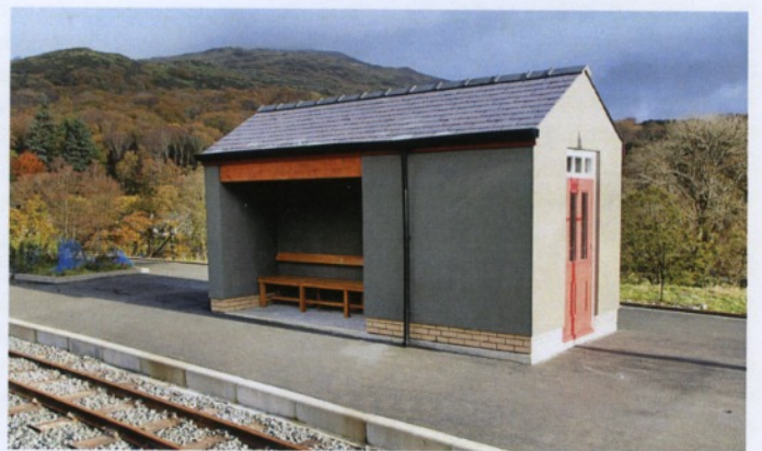
Beddgelert station shelter - 2008 style - David Allan November 2008
