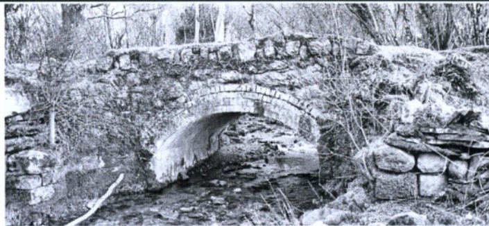
Arched river bridge at Bicall, north of Tryfan Jct
