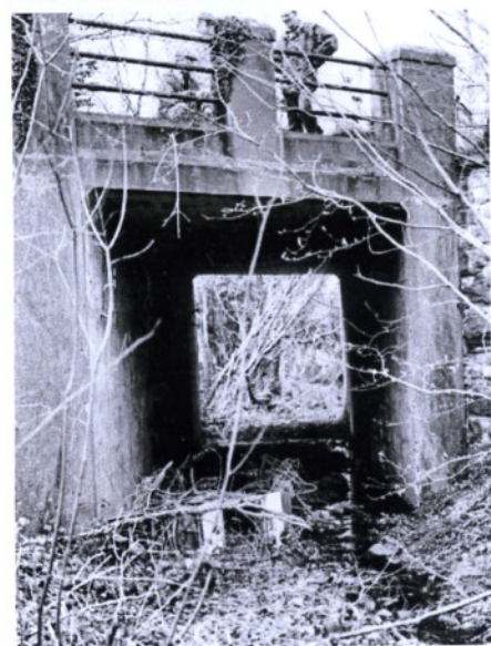
Wernlas Ddu road bridge
