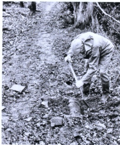
Exposing the earthenware water supply pipe
