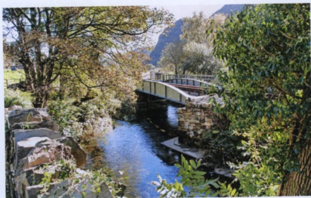
Bridge over the Afon Gwyrffai at Plas y Nant
