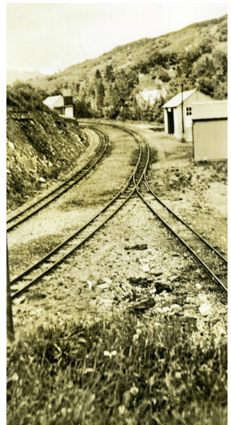
Top - Beddgelert Siding - note Croesor chairs. Above - Beddgelert station & bookstall
