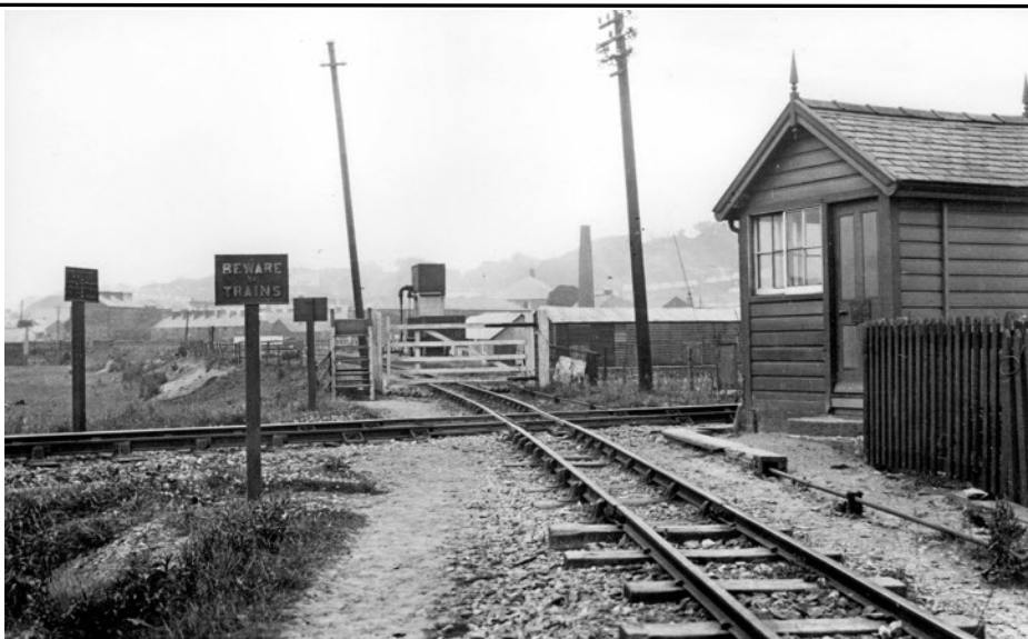
Photo 6: The transition from ex-standard gauge bullhead to W.H.R. shows a marked change in rail section. Note the higher position of the W.H.R. sleepers on the bed of ballast, and the cranked fishplates to accommodate the difference in height and cross section. The point rodding runs both north and south of the crossing; bullhead rails run under the gate to the south, so was the trap point constructed from bullhead materials?
