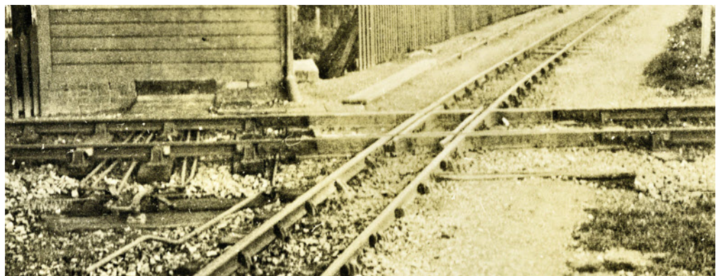
Photo 2: An enlargement of part of the "Antia" photograph indicating features referred to by David Smith such as; the lighter coloured, slab-sided rails on the crossing itself, consistent with it being manganese steel, and the very short WHR crossing rail stubs.
