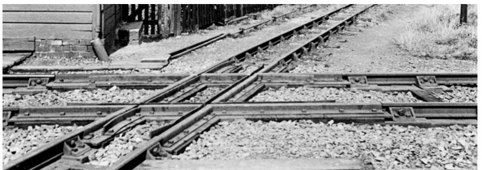
Photo 5: A close-up of the post-1928 crossing in bridge rail, showing features such as (a) 1" oak packing on the longitudinal timber baulks (b) Rails and angle irons bolted down (c). Special through-bolted chairs for the bullhead transition on timber baulks.
