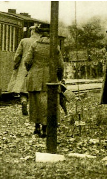
Above right - an enlargement of the top of the pole at Snowdon station showing the insulators mounted on brackets, but no wires, and the possible lightning conductor. There appear to be other clamps mounted on the post possibly for electrification anchor cables, or mounting brackets for the cable support arms. Left - the foot of the pole showing the parallel section and the ‘ring’ or ‘boss’, plus tensioner for the ‘guy’ cable.
