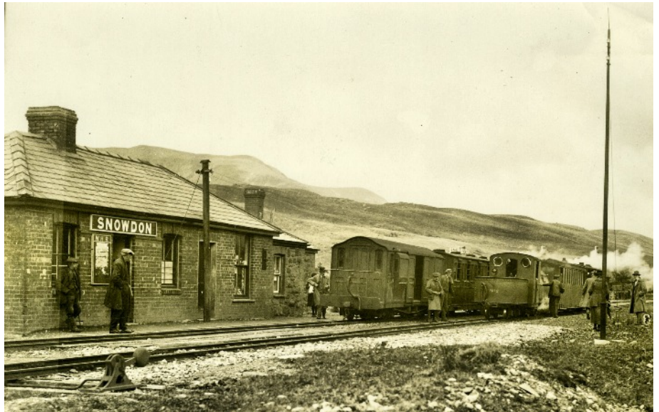
The photograph taken in early WHR days at ‘Snowdon’ station, before it was renamed ‘South Snowdon’. One of the tall metal posts is clearly visible on the right hand side, with a supporting guy cable. There are two insulators mounted above one another towards the top, and what appears to be a lightning conductor atop the post. A conventional timber telegraph pole is in place alongside the station building; this was erected some years previously and appears in older photographs. The shape of the insulators suggests that this could have been an electricity supply pole, but lurking behind the visible insulators on the cross piece are two more, of the typical ‘telephone’ shape. Indeed twin phone wire can just be made out leading away from the pole..
