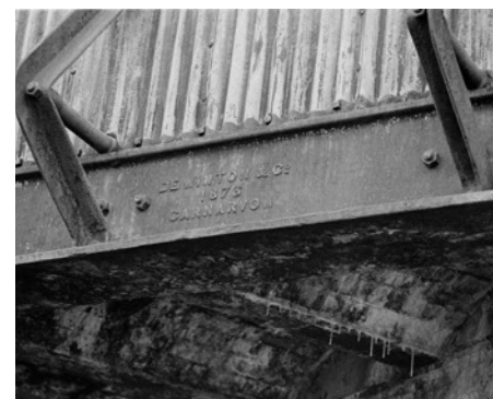
One of de Winton's surviving bridge beams - from the road over bridge near Betws Garmon Station on the N.W.N.G.R.
