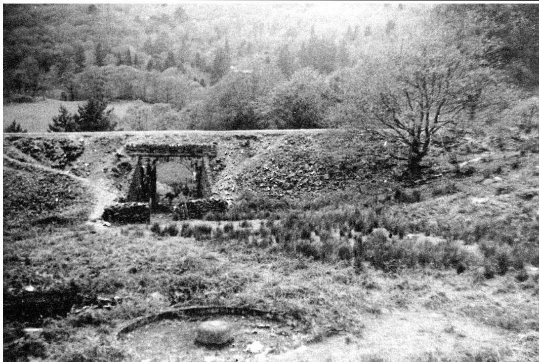
Figure 3. Bridge through W.H.R. embankment, with circular buddle in foreground. (Gwynedd Archive Services)
