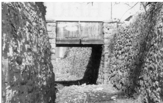
N.W.N.G.R. Track passed through Rhostryfan in a cutting - the girder bridge carried the 'High Street' over the railway. Bill Rear 1948.
