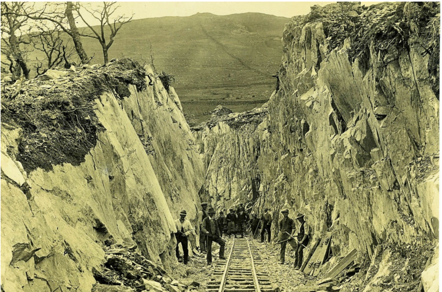
Excavation of the ‘new’ deep cutting above Beddgelert on the re-aligned Welsh Highland route - Williams - ca. 1922
