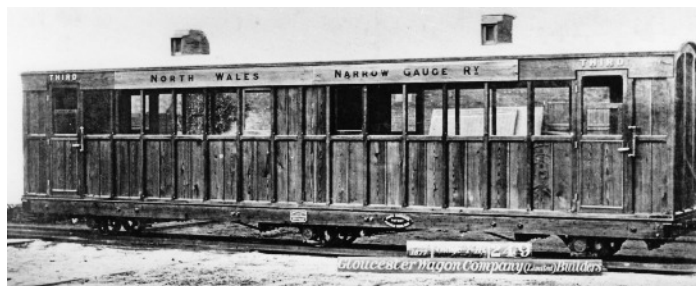
Russell's purchases included the Railway's three Cleminson 6-wheel carriages Nos. 6, 7 and 8. The three comprised one All-3rd Saloon and two Brake/2nd/3rd Composites - WHR 186 (left) and WHR 187 (right)
