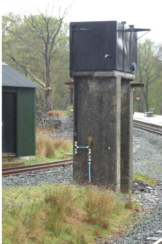
A view of the 'main line' and 'south' elevations of the Beddgelert water tower - note the bag support bracket, the discharge at the top end of the tank and the pipe work described in the text Peter Liddell (May 2015)
