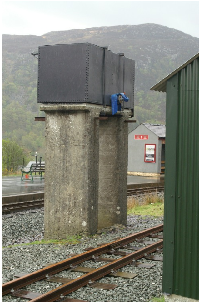
The ‘lamp hut’ and ‘north’ elevations of the Beddgelert Water Tower - note the location of the outlet on this side of the tank, discussed at some length in the text - Peter Liddell (May 2015)
