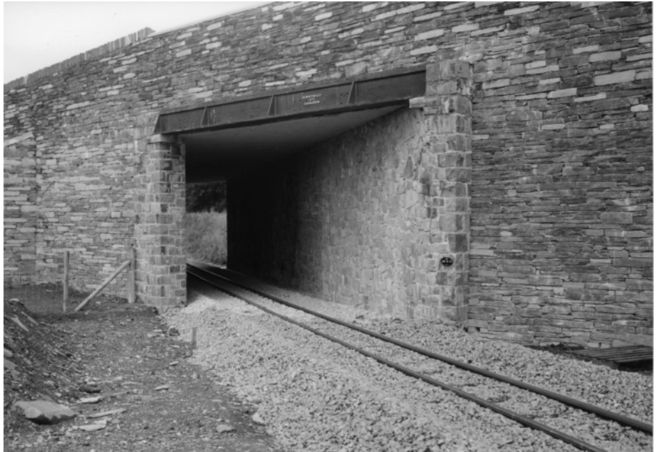
The De Winton beams from the original Bettws Garmon road bridge preserved in today's rebuilt bridge. The original makers name and the date of 1873 have been highlighted during reconstruction. (David Allan - 2003)
