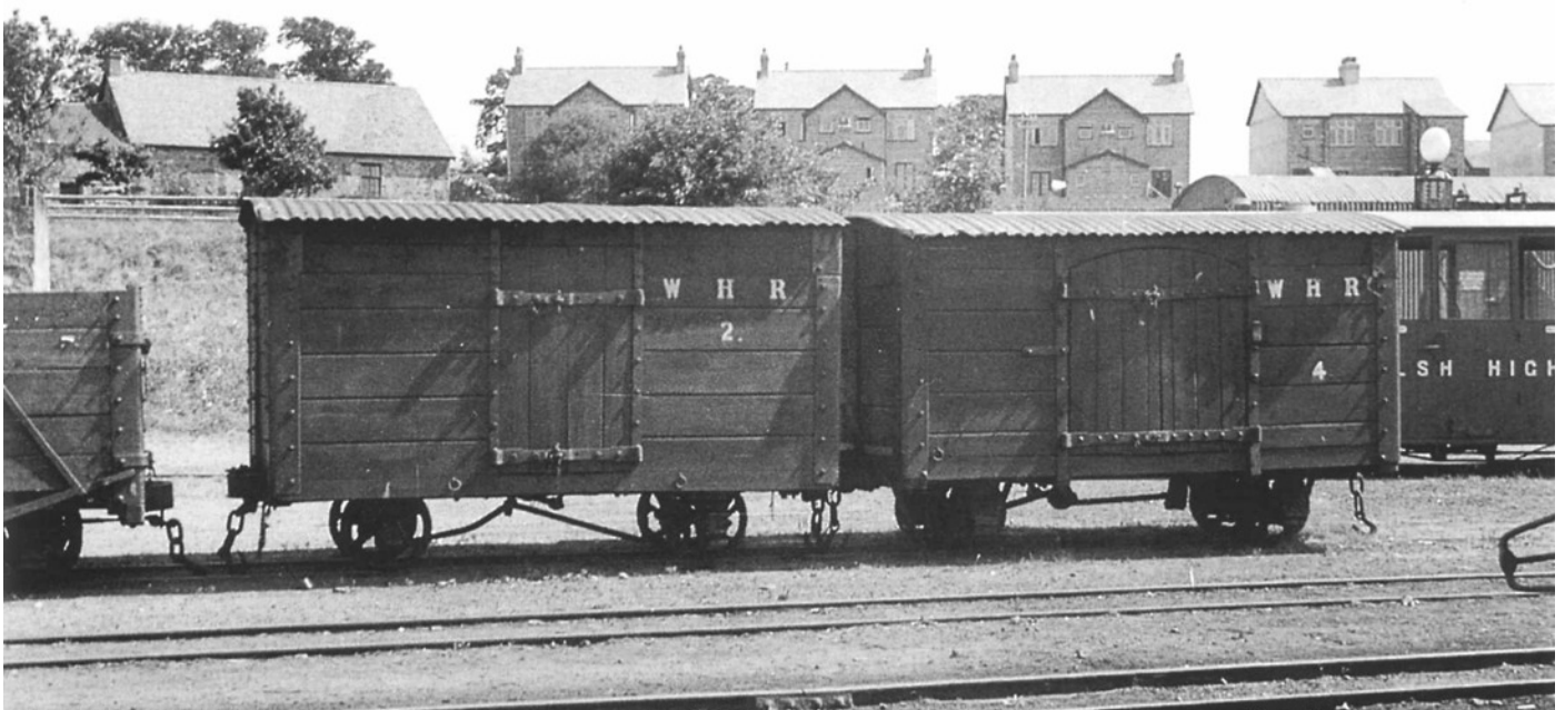
Both of the Welsh Highland Covered Vans photographed at Dinas Junction by Hubert Wheeler on August 8 th 1935. Note the completely different approaches to door design adopted for No 2 and No 4 as discussed by Stuart in his letter above. Note also the differences in brake mechanism design to which he refers and how the wheels and brakes on No. 2 appear 'lighter' than those on No. 4
