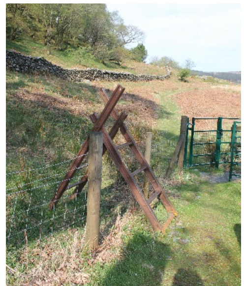
The two stiles at Salem described by Lewis Esposito in his notes on Page 3. The photographs show the new 'gate' stiles installed by Gwynedd County Council and the National Park with the reinstated NWNCR rail-built stiles alongside.
