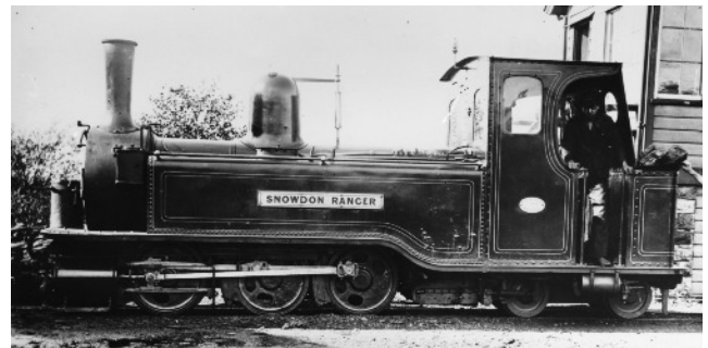
Figure 1 (left) - Maker's photo of Snowdon Ranger 1875 - note sand-box arrangement, whistle location and maker's plate. (WHR16)
