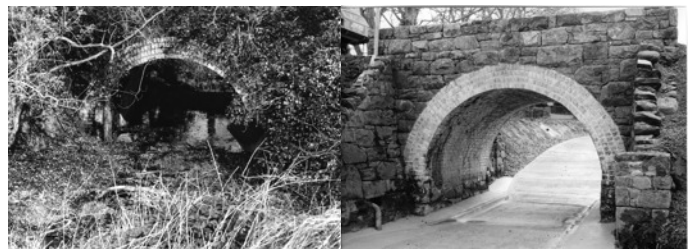
The occupation under bridge at Bod Aden, before (1998) and after (2000) rebuilding (UB10) - David Allan.
