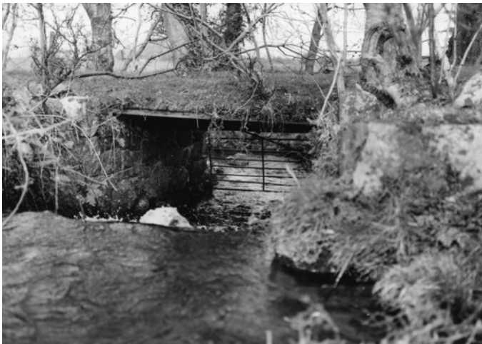
The girder- and rail-built bridge over the Afon Rhyd near Bod Aden - since fully re-built, this is today's UB12 - David Allan.
