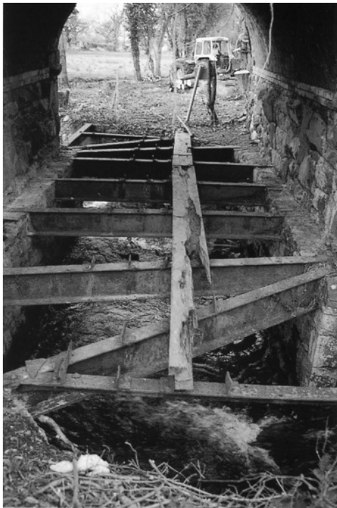
The road over bridge at Cae Moel as it was, showing the girders that had carried the track above the Afon Rhyd
