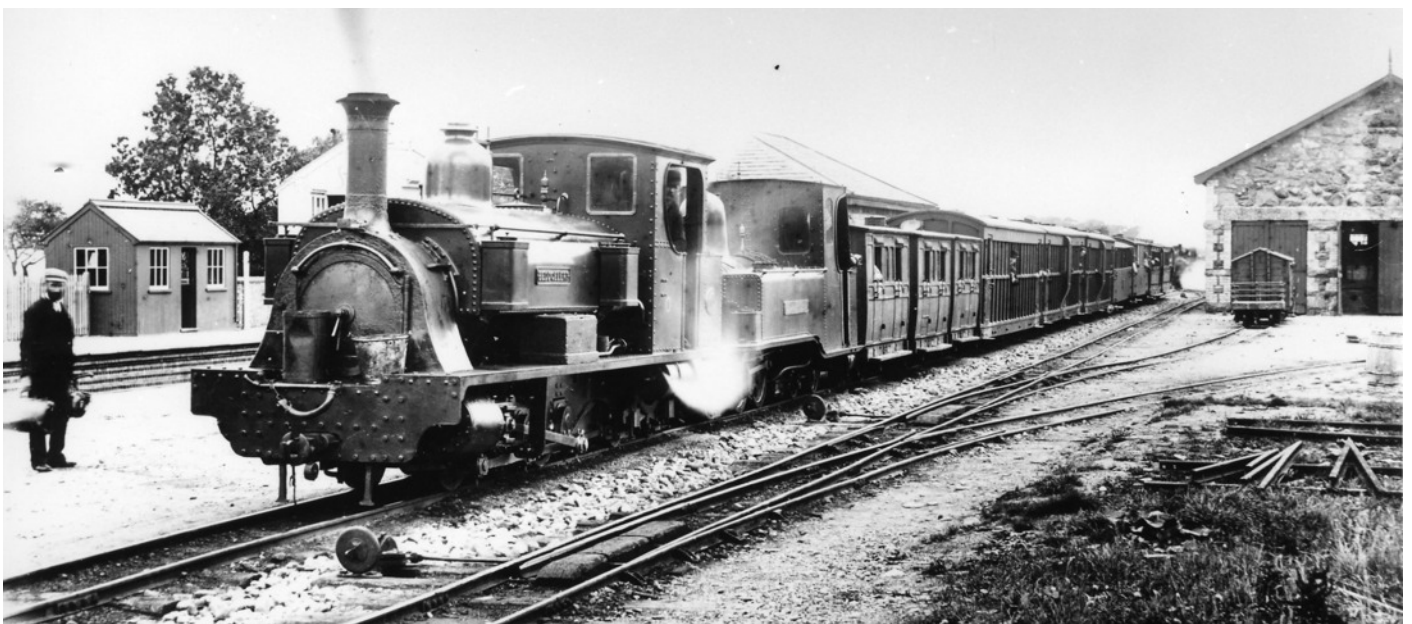
Beddgelert and Snowdon Ranger with all the NWNCR carriage stock acquired by the railway up to and including 1891. The train comprised the three Ashbury 4-wheelers (running together), the all-3 rd Cleminson, the two Cleminson Brakes, the Workmans and Tourist Cars from Metropolitan and both Ashbury Brake composites. A third locomotive, presumably Moel Tryfan, can be seen beyond the rear of the train.
