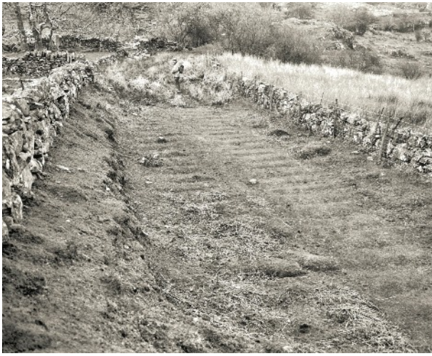
Figure 1 - Site of 1890's transhipment wharf. Sleeper marks of wharf siding on left, with those of the main line on the right. D.W. Allan. 2000.
