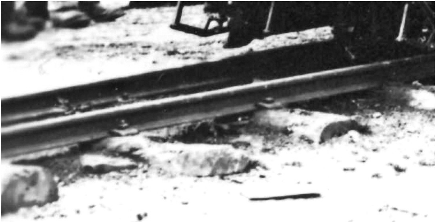
Figure 1 - Original NWNGR track-work at Rhyd-ddu ca. 1892. Note the use of logs as sleepers, the method of attaching the rails to the sleepers and the indifferent alignment of rail levels. At this time there was no passing loop here and train reversal - this was the terminus of the line - would have been 'interesting'. WHR 1093
