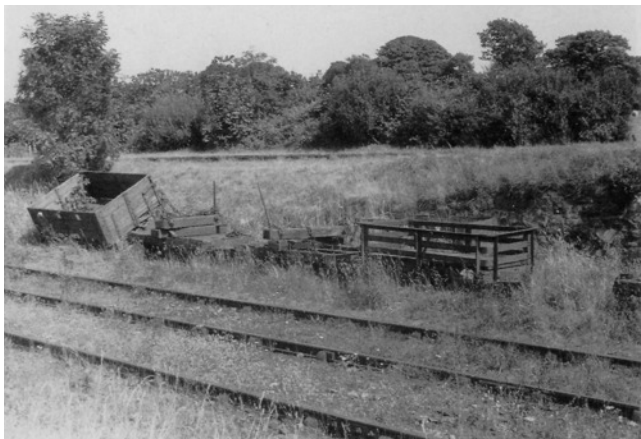
Above left - beyond the slate wagon, two of the 'tipping' wagons sit at Dinas in a train of disused stock parked on the carriage shed access line - note that their opening doors are on opposite sides - J.F. Bolton October 1941 - WHR 77.
