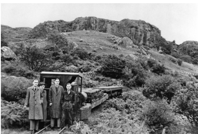
Cohen's Demolition Train to the south of Glanrafon Sidings. J. F. Bolton - 1941 - WHR 83
