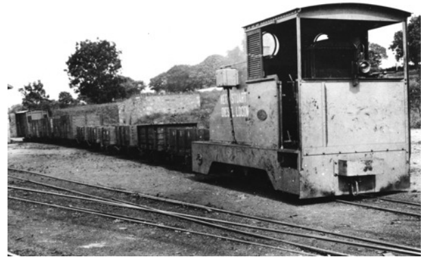
4415 with a goods train about to depart Dinas in 1928 - Arch 3625.
