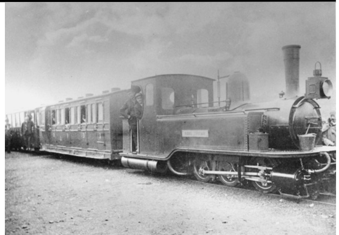
Moel Tryfan and train awaiting the arrival of Sir William Gladstone, Dinas, 12 th September 1892 - Arch 3622
