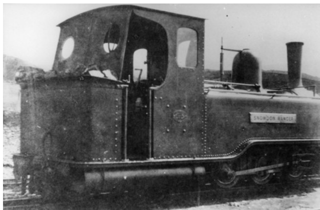
Snowdon Ranger with maker's plates fitted (the plate shows that the boiler was still original) and high-level sand box installation - Arch 3306
